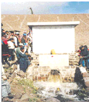
Left: Construction of Reservoir in Pisac (Peru, 1999)
